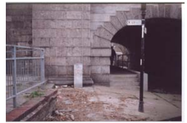
Connections under Kew Bridge should be enhanced
