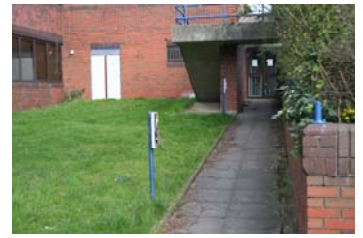
Connections between Waterman’s Arts Centre and the Thames Path towards Ferry Quays need to be made legible and welcoming
